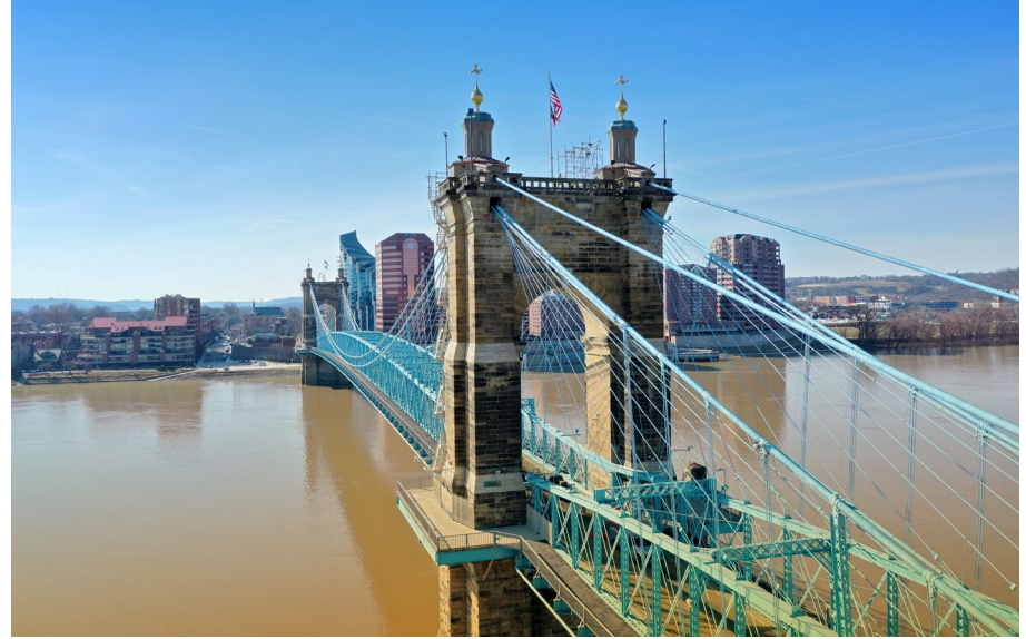
John A. Roebling Bridge Cincinnati, OH
