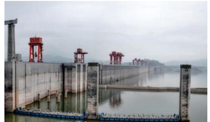
Three Gorges Dam, China
