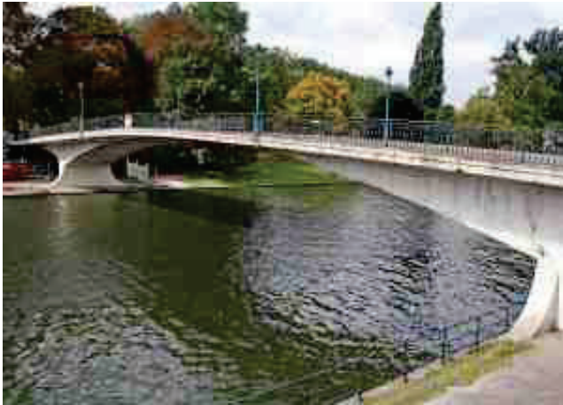
Arch bridge at Châtelleraut, France, 1899, Francois Hannebique -1905, Engineer and builder, who patented reinforced-concrete construction in 1892.
